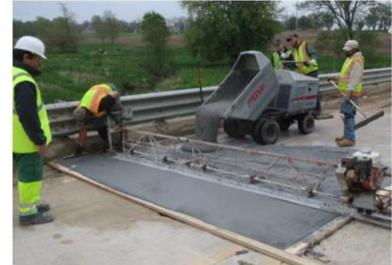
床版の上面増し厚補強 (B. Graybeal et al.: International Perspective on UHPC in Bridge Engineering, 2020)
