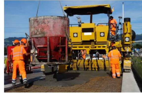
床版の上面増し厚補強 (B. Graybeal et al.: International Perspective on UHPC in Bridge Engineering, 2020)
