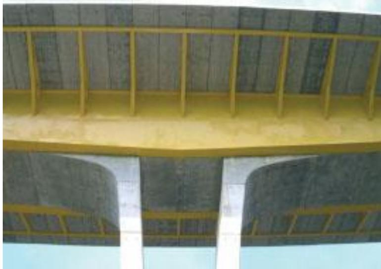
*Fig. 15. View of the rigid connection between main pier and steel deck*
