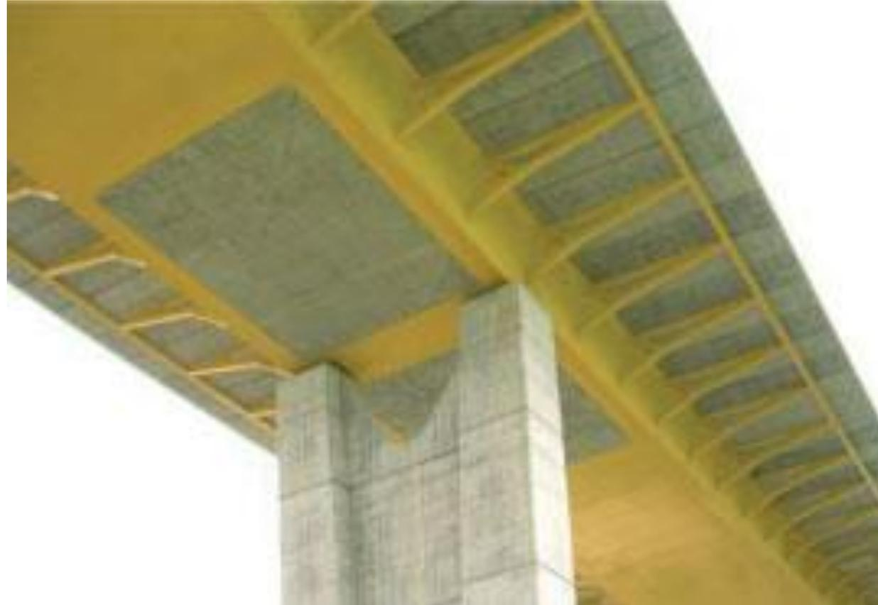
*Fig. 5. Hogging bending moment zone with double composite action*
